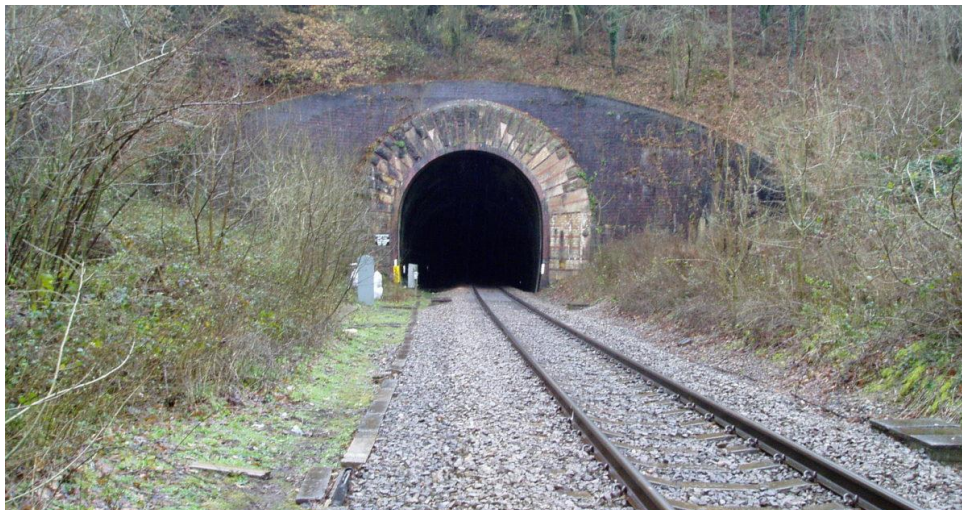
Figur 3-1 Enkelt sporet jernbanetunnel (Chipping Campden tunnel, England)
